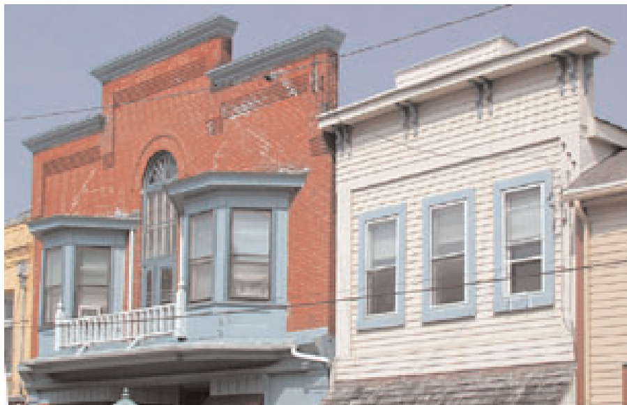
Side-by-side examples of brick and frame upper facades on Main Street. Both have parapets (walls that project above the roofline) with decorative features – corbelled brick on the left and wood brackets on the right. The brick example also has a decorative 2nd story, including projecting bay windows, a round-arched window and door with balcony.
