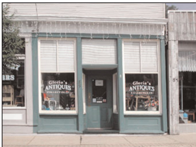
A traditional storefront with evenly spaced openings. Two display windows flank a recessed entry door.
