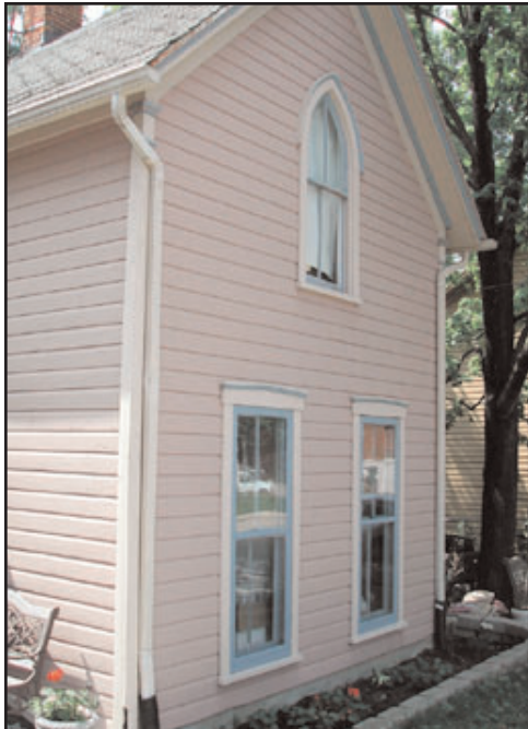
Waynesville example of beveled wood siding, wood corner boards and wood window trim that is kept painted and well maintained
