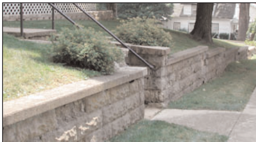
Examples of concrete block and limestone retaining walls.
