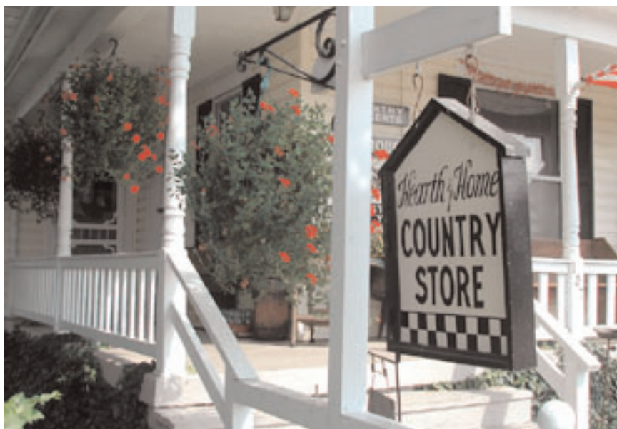
The original residential character of this building is still evident
