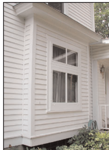
A wood storm window that reflects the design of the window behind it
