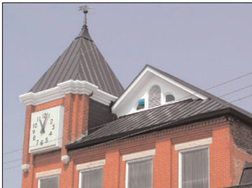
The Waynesville National Bank's roof was replaced with a new standing-seam metal roof in recent years. Care was taken to maintain the weather-vane finial on the tower and other details of the roofline.
