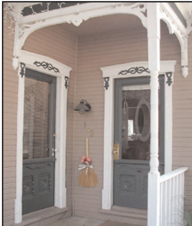
An example of a pair of doors set into an angle of the building, found on a gabled cottage
